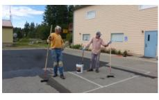
Center parking lot. Ski and Ray carefully filled in all the cracks, added sealer, and painted court lines on making it a much improved surface.
